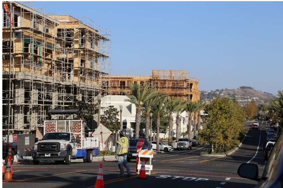
New housing being constructed in the Town Center in 2020
